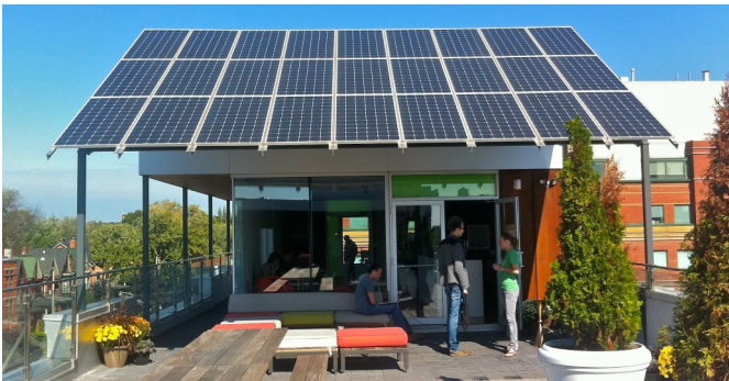
Solar Panels Integrated with Building Design
